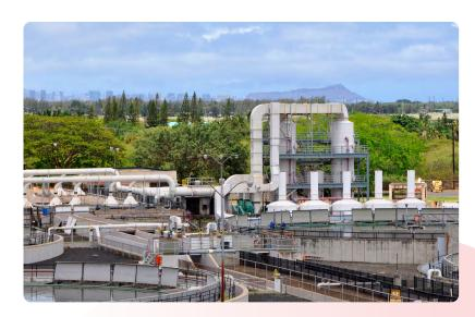
Veolia North America partners with a wastewater recycling facility in Honolulu, Hawaii, which recycles nearly 12 million gallons of water a day — using reverse osmosis and UV disinfection to treat the water. The facility can hold nearly 13 million gallons of secondary effluent per day, which is used to power industries and irrigate nearby landscape.
